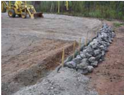
Dike installation for oil and rainfall requirements.
