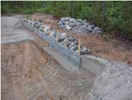
Water gate install to process water.
