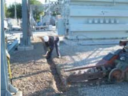
Dike installation for oil and rainfall requirements.
