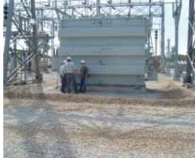
Dike installation for oil and rainfall requirements.
