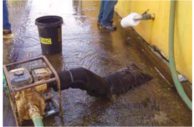
EVAC filters water from concrete containment.
