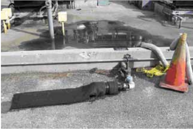
EVAC filters water from concrete containment.
