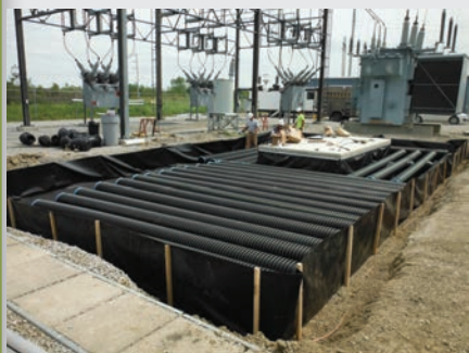
Geomembrane Liner System with Oil Filtration Panels uses HDPE corrugated pipe to accommodate a smaller footprint.
