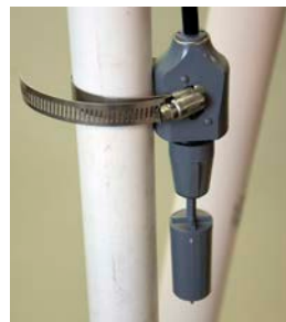
SCADA High-Level Alarm (left) warns of high water or a malfunctioning pump
