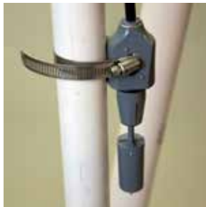
SCADA High-Level Alarm
