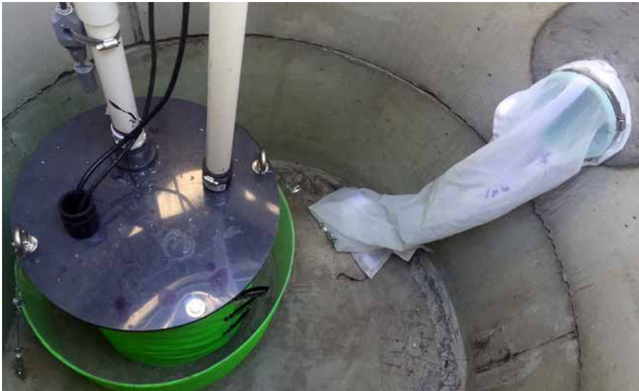
Completed VIPOR System installation for substation containment
