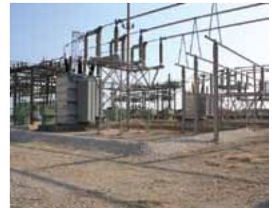
SPCC compliant containment in one day.
