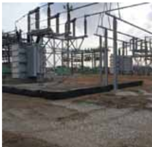
C.I.Agent ® Barrier Boom staked in place.
