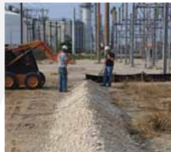
Workers rake the finishing touches on the dike.
