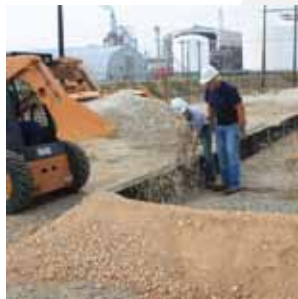
An angle iron is held in place over the Barrier Boom while gravel is poured on both sides of the Boom.
