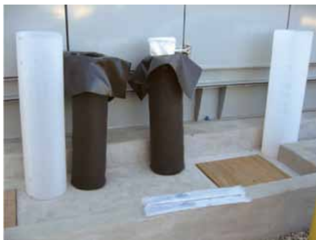
C.I.Agent® Hydrocarbon Flow Filters, white pre-filter and outer cores next to installation holes (covered by plywood).
