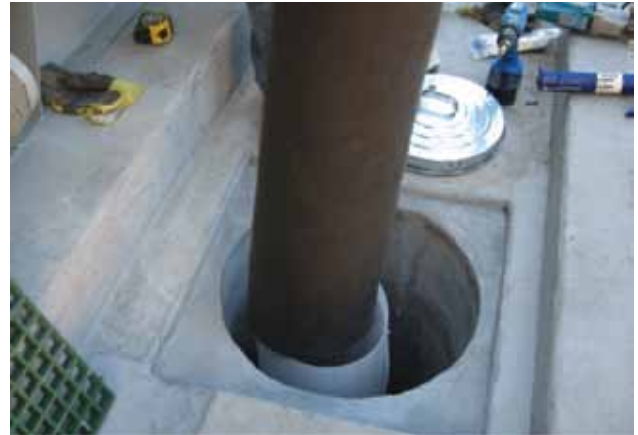
The Hydrocarbon Flow Filter is slid into the outer core.
