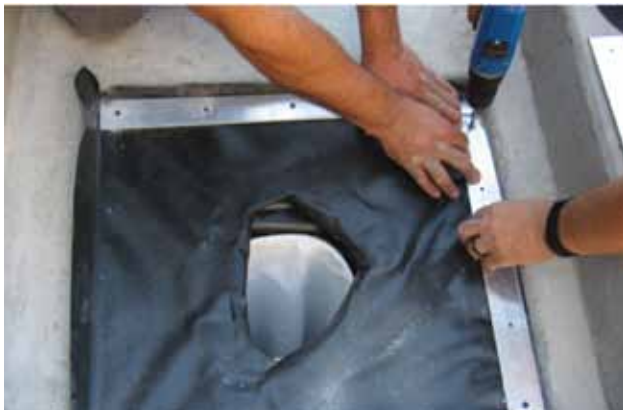
Aluminium strips screwed into the concrete ensures the seal.
