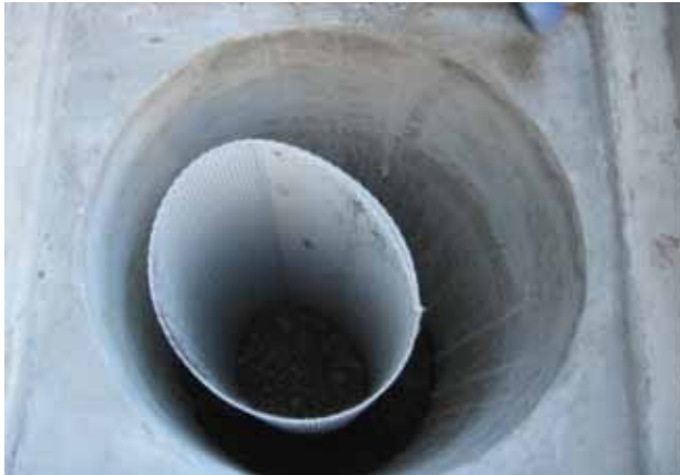
Gravel poured to support outer core and Hydrocarbon Flow Filter.
