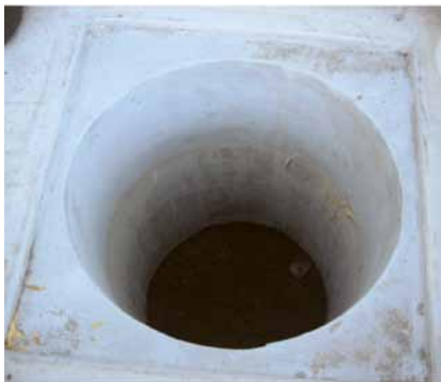
Containment area hole ready for Hydrocarbon Flow Filter installation.
