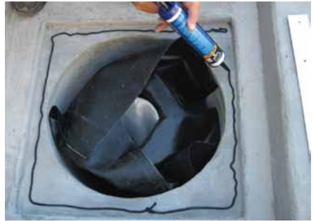
Sealant is applied to concrete to secure the flange.
