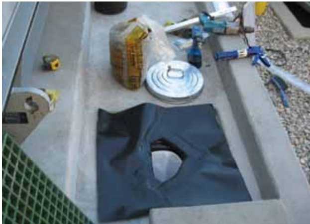
Vinyl flange is put into place and checked for fit.
