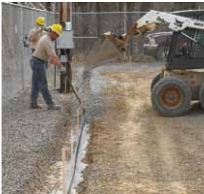
7. Stakes are trimmed off to ground level. Carefully dump clean stone in the trench and around the Barrier Boom being careful not to crush the boom. If using rebar, pull it out of the ground once clean stone is around the boom.
