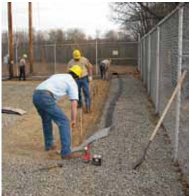
4. Position stakes or rebar every 10 feet inside the trench. Roll out the C.I.Agent® Barrier Boom beside trench. The BLACK fabric side of the Barrier Boom must be up.
