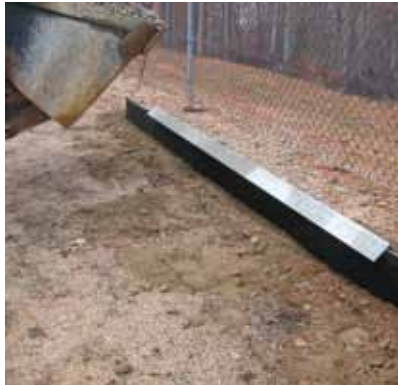
8. A 10 foot angle iron can be used to deflect the stone during the fill process. Rest the angle iron on the stakes or rebar and pull the angle iron to the next support during filling.
