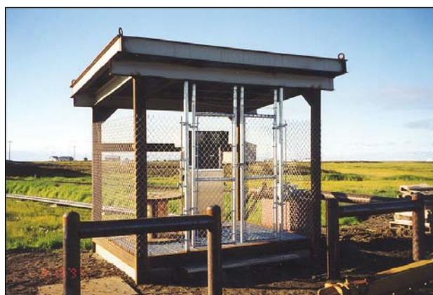
**Figure 3-2.** Fencing around a dispenser pump.
